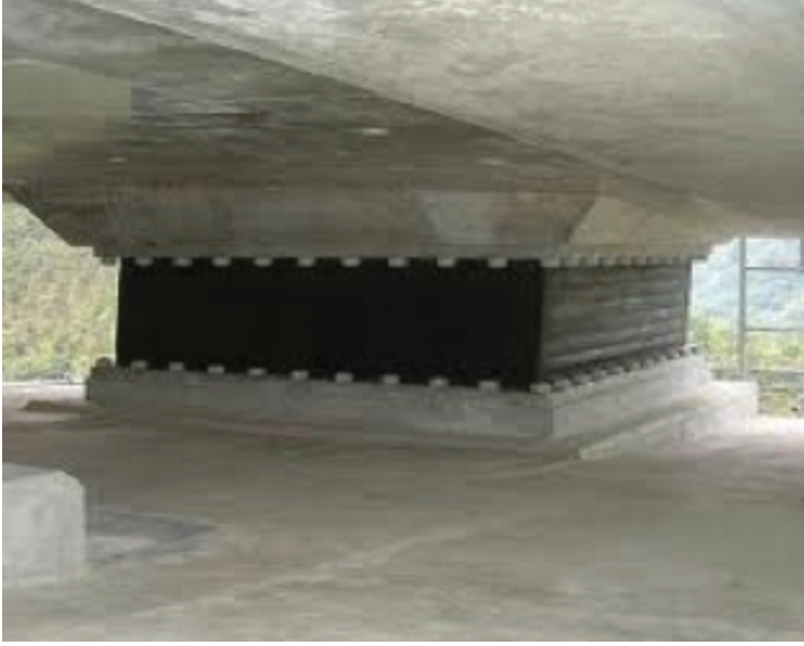
Çelik Plaka takviyeli Kauçuk Mesnetler / Reinforced rubber bearings with steel plates
